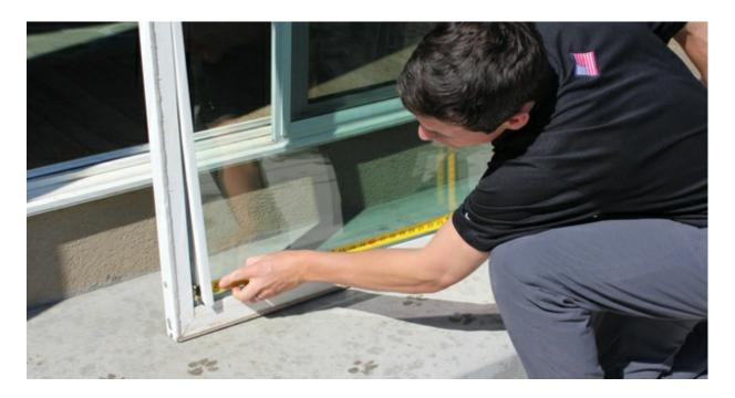
Step 2. Separate Glazing Tape Between the Frame and Glass.
