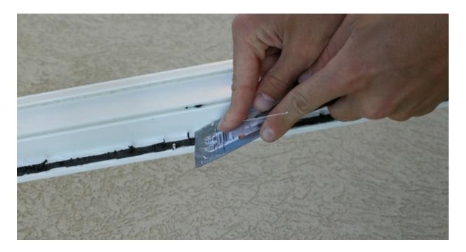
Step 4. Apply Fresh Glazing Tape on the Door Frame.
