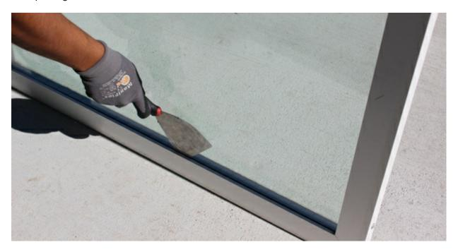
Step 3. Remove Old Glazing Tape from the Door Frame.
